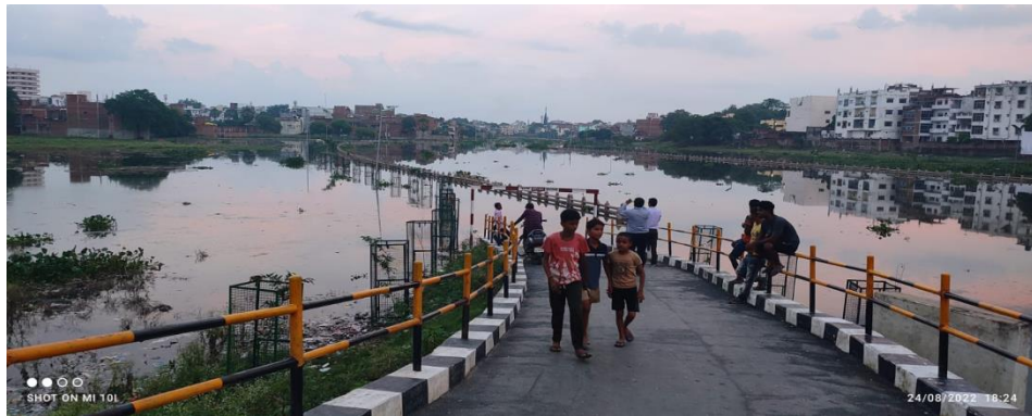
Corridor submerged in Flood Water of River Varuna
